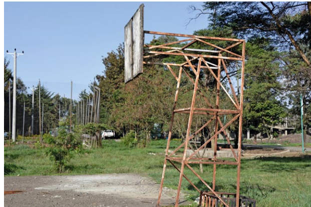
Typical bending, aging, fading out of colour; incorrect dimension and corrosion problems on goal and basketball post installations.
